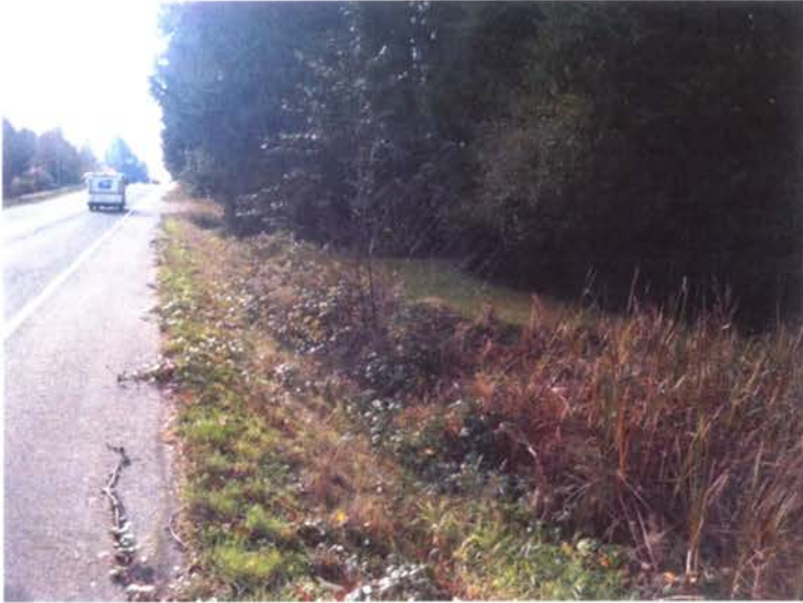
Photo I: Looking south at unmaintained drainage ditch that slopes down to the north.
